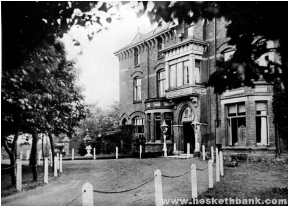
Figure 6. Photograph dated 1912, showing the front elevation from the north east ( ://www.heskethbank.com/history/photos/pubs.html )
